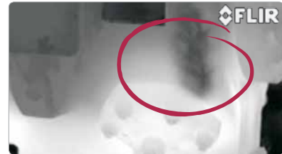
Captured gas leak.
